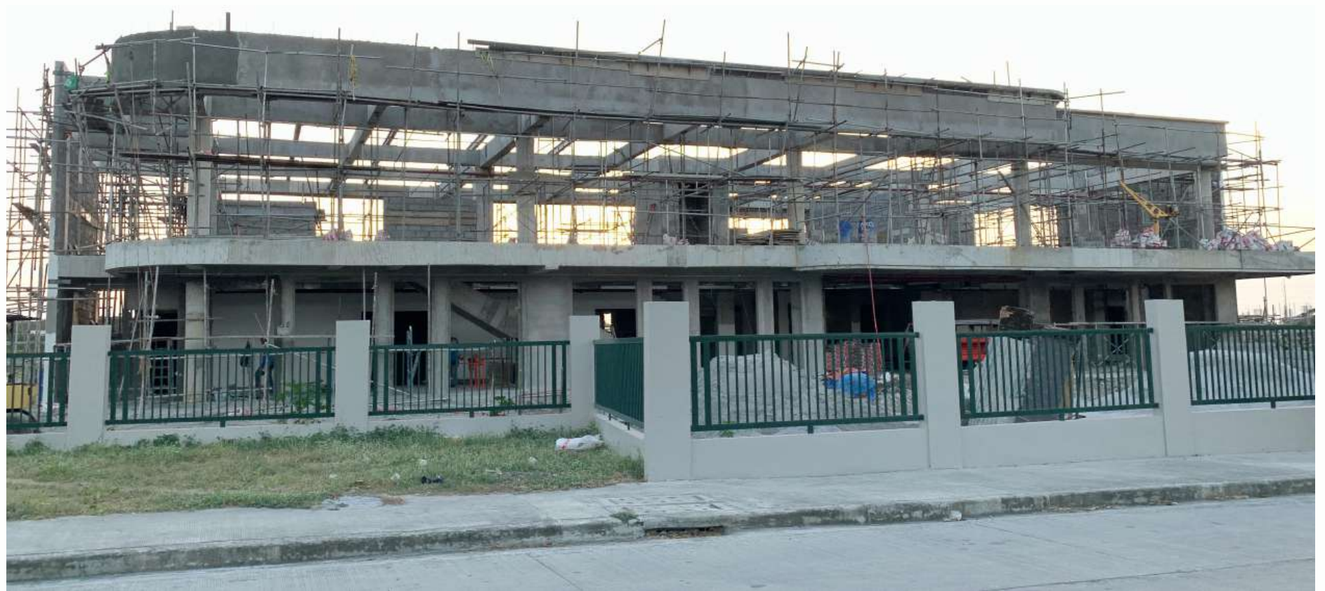
The On-going Construction of the Museum of the Human Body
