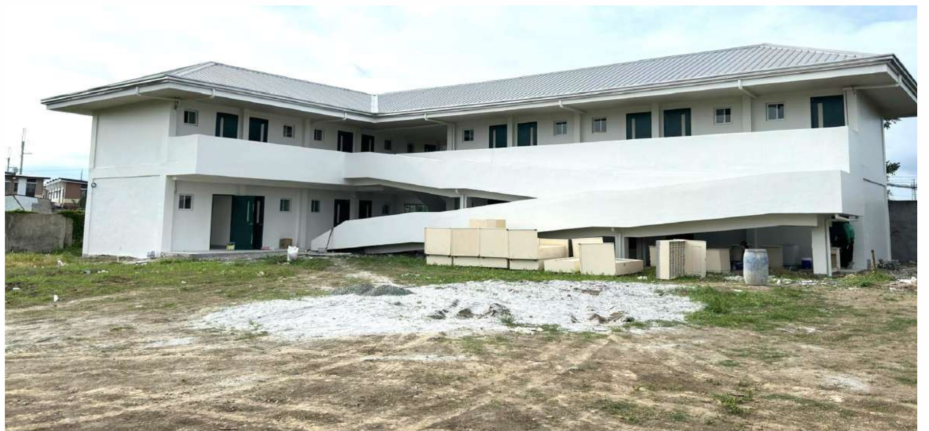
The Isolation Facility
